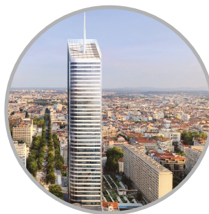
Distech Controls SAS European Head Office Lyon, France
